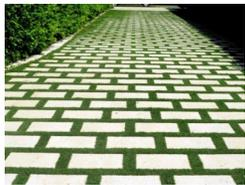
**Permeable Paving:** Constructed from a range of sustainable materials and using many different techniques, permeable pavements generally consist of a base such as bare soil or a seeded ground-cover overlaid with bricks or another porous yet sturdy material that allows the movement of stormwater through the surface. In addition to reducing runoff, this effectively traps suspended solids and filters pollutants from the water.
