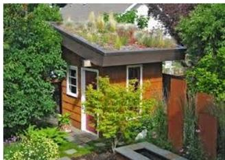
**Green Roof:** A green roof is a conventional roof that additionally supports a waterproof membrane, a growing medium and soils that support living vegetation. Also known as living roofs, vegetated roofs, or eco roofs, these systems are usually planted with perennial, self-sustaining and drought resistant plants to minimize maintenance. Proper consultation with a professional is recommended to ensure roof stability and system success.
